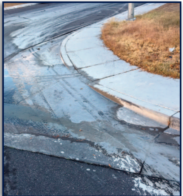
Litter, pollutants and concrete washout in the streets, enter nearby storm drains and get carried untreated to Lake Mead.
