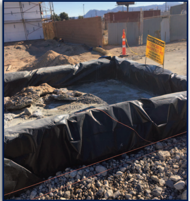
A well-maintained concrete washout area.
